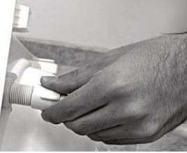
If the faucet has been installed over the washbasin, a flexible hose (not included) is necessary to connect the faucet to the water supply. Screw the flexible hose to the faucet first; after you have fixed the GabFit, connect the flexible hose to the water supply. We recommend the use of Astra's flexible hoses.
